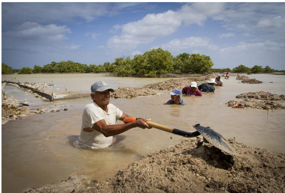
Figure 3. Construction of the channels through manual excavation Sodzil community.
